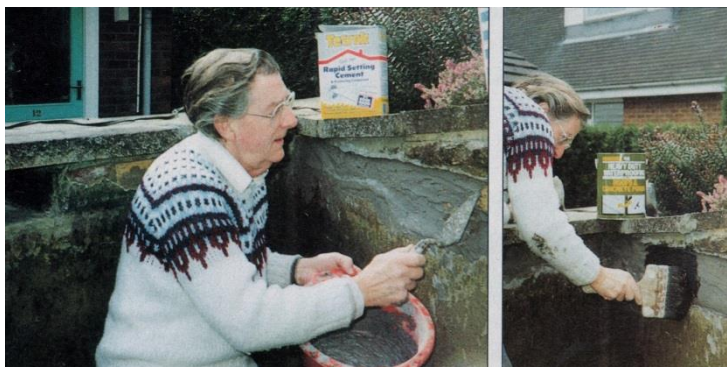
Use rapid setting cement to fill cracks and seal with pond varnish
